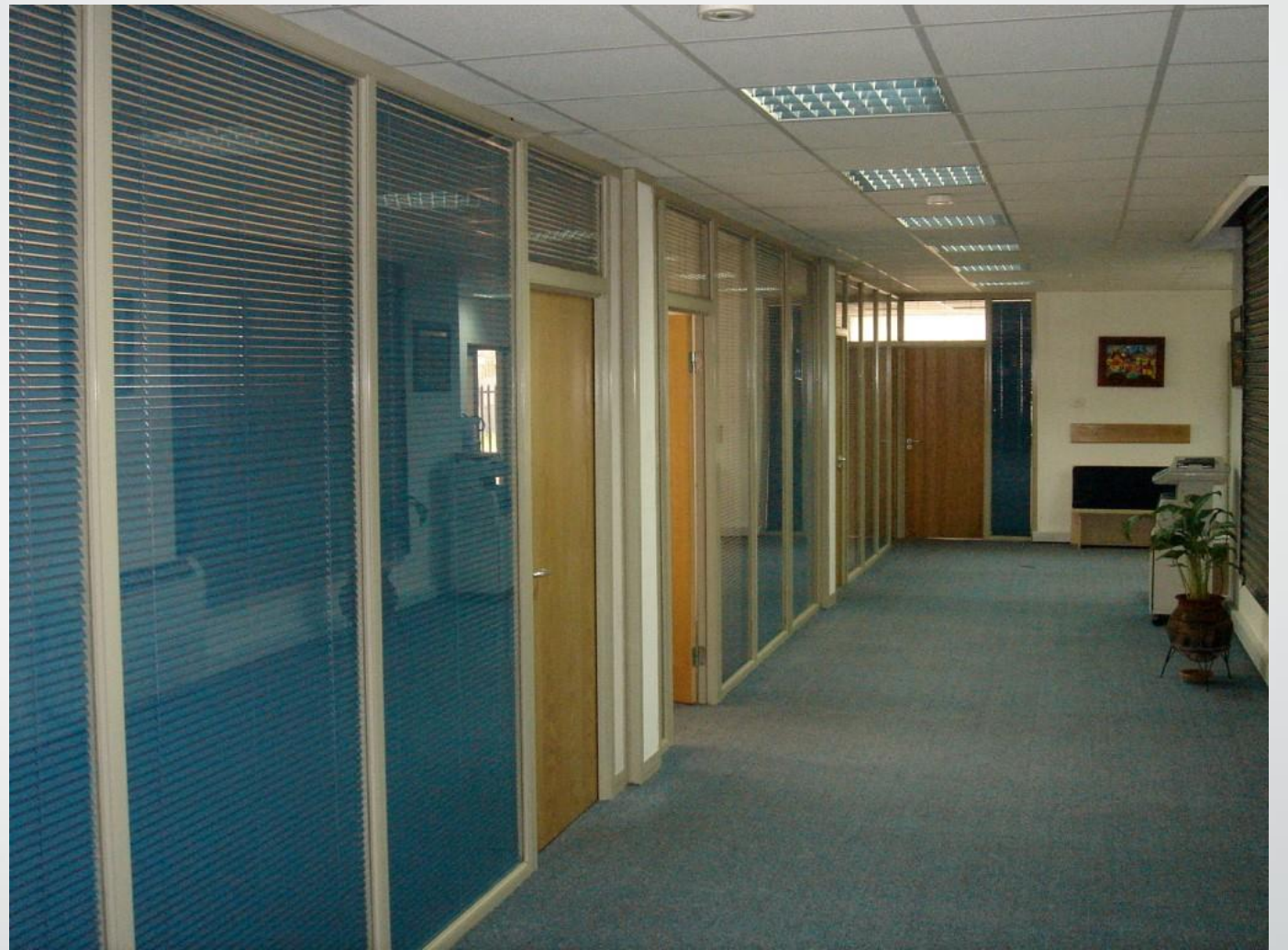
Framed glass partitioning
